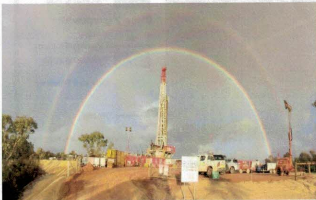
Figure 2. Waitsia-3 Appraisal Well drilling, July 2017
